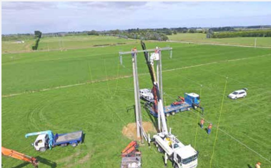
PowerNet Field teams replacing a two pole structure on the North Makarewa to Winton 66kV line
