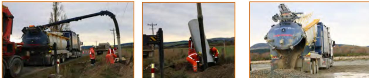
L-R: Skevington's vacuum truck extracts gravel from the holes before inserting the steel liner to prevent hole collapse.
