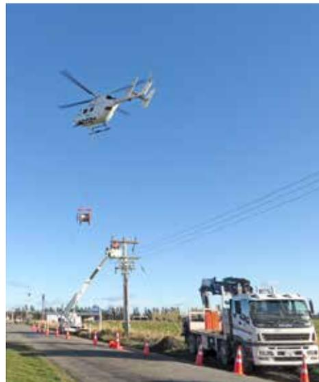
Staff from Otago Power Services installing the 66kV conductor on the new 66kV line
