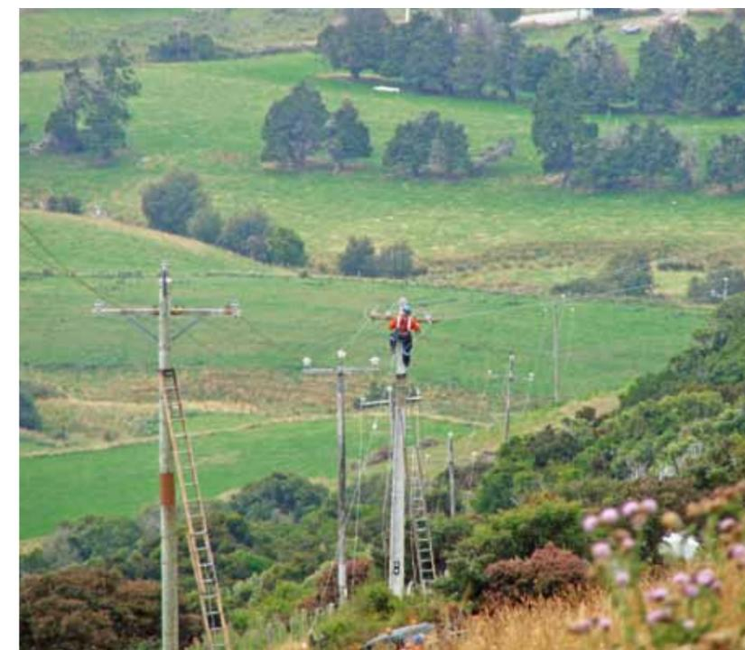
Otago Power Services line mechanic working on pole replacement on the Owaka to Tahakopa 11kV line
