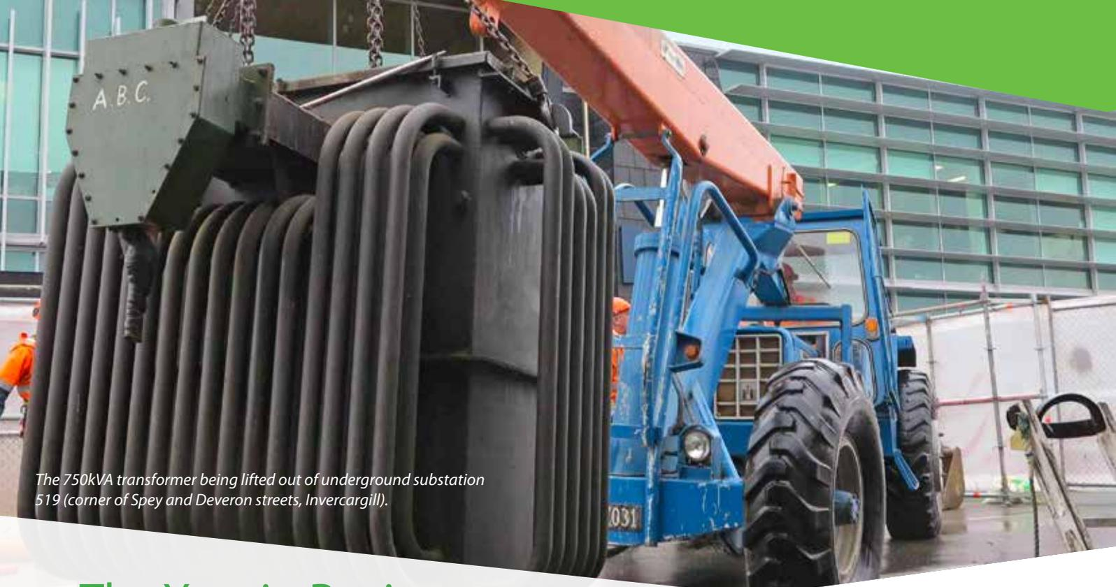
*The 750kVA transformer being lifted out of underground substation 519 (corner of Spey and Deveron streets, Invercargill).*
