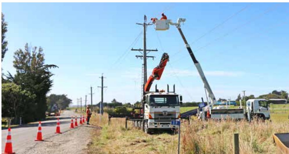
Pole replacement at Makarewa
