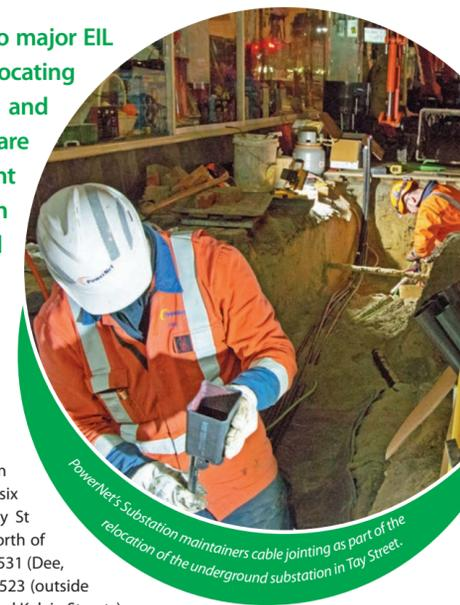
PowerNet's Substation maintainers cable jointing as part of the relocation of the underground substation in Tay Street.
