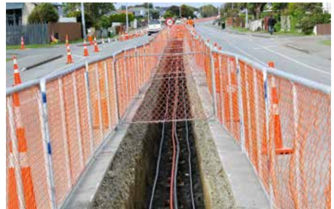
Stage 2 cables pull on Yarrow Street
