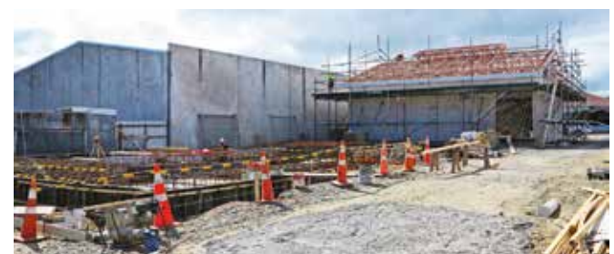
Spey Street Substation under construction
