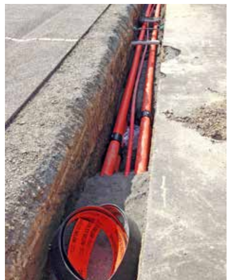
Ducting laid in Jed Street
