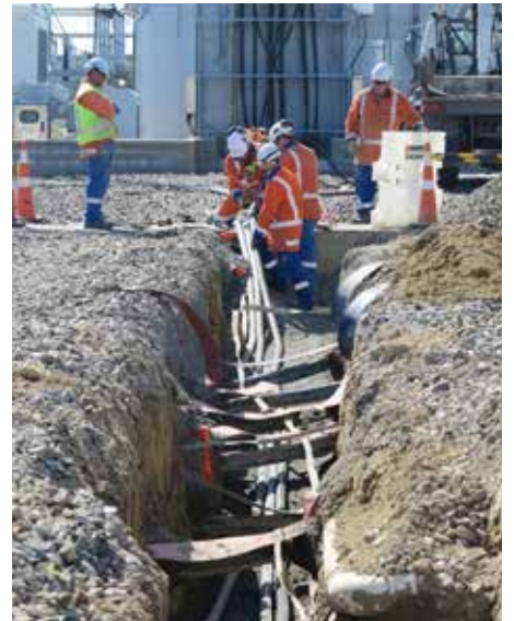
Staff from Electrix, Bond Contracts and Delta installing the 33kV cable to the Transpower grid exit point in Invercargill
