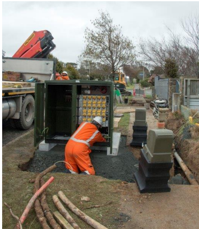
Transformer Replacement Metzger Street, Invercargill
