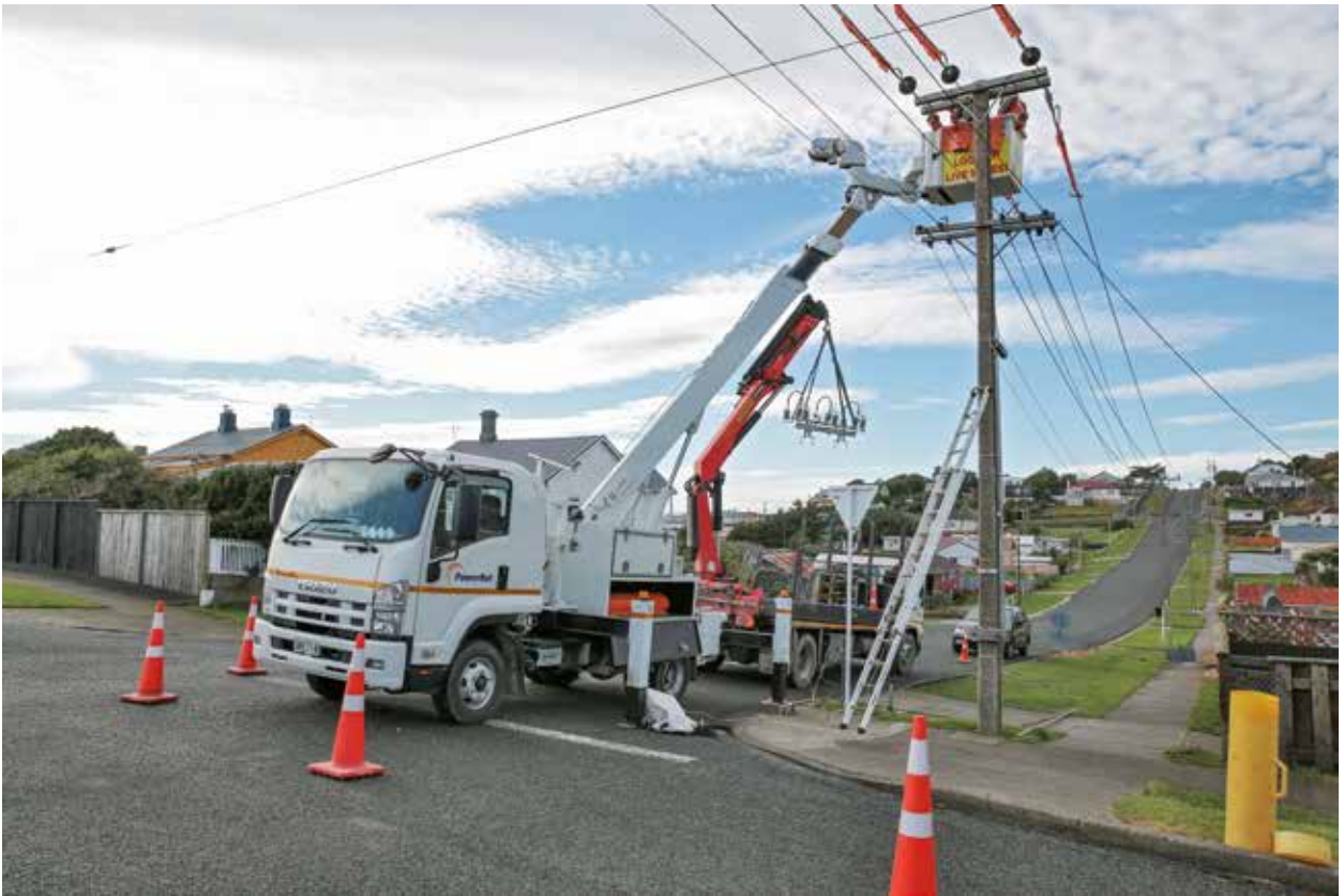
PowerNet field maintenance team working on the Electricity Invercargill network in Bluff
