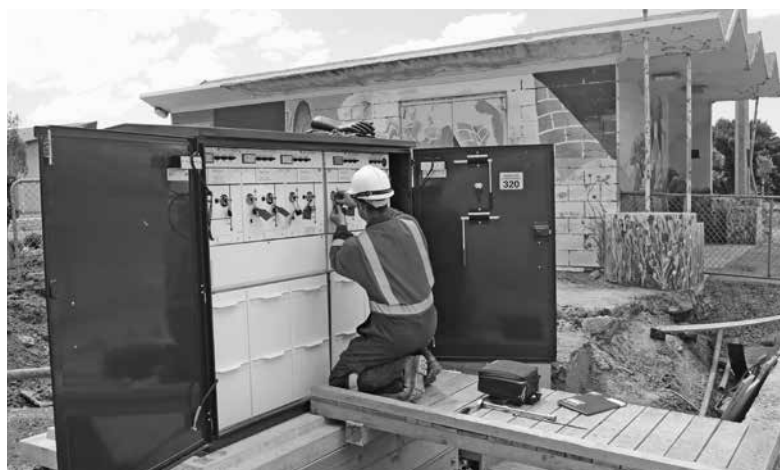
Jason Nicolson (PowerNet) working on the Ring Main Unit at the Glengarry Shopping Centre.
