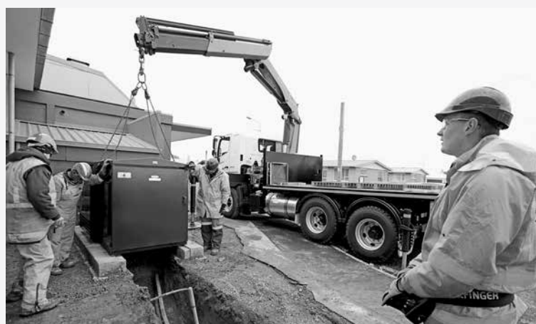
Staff from PowerNet and Bond Contracts placing the 750kVA transformer on site at Windsor New World
