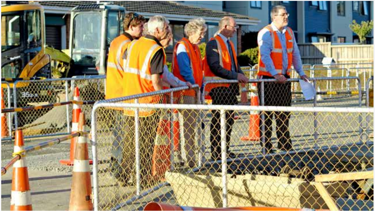
Above and below: Upper Spey Street residents viewing the Spey Street Substation
