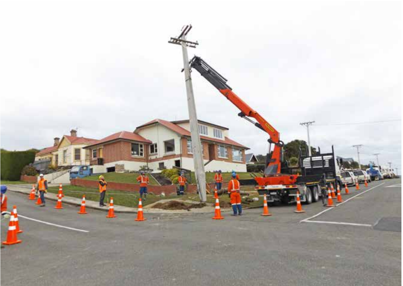
Pole replacement in Bluff township
