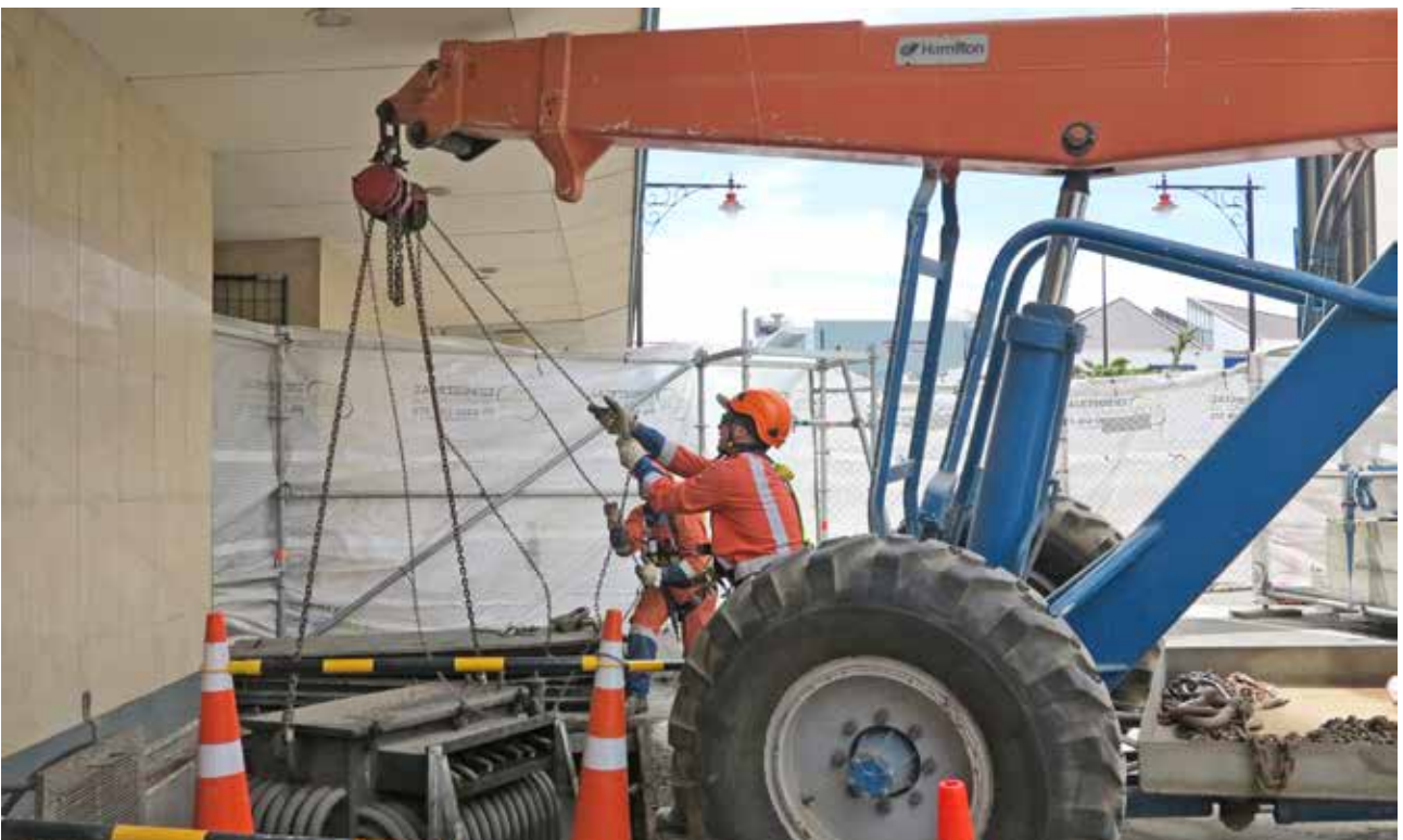
Decommissioning of the underground substation outside the entrance of the Kelvin Hotel
