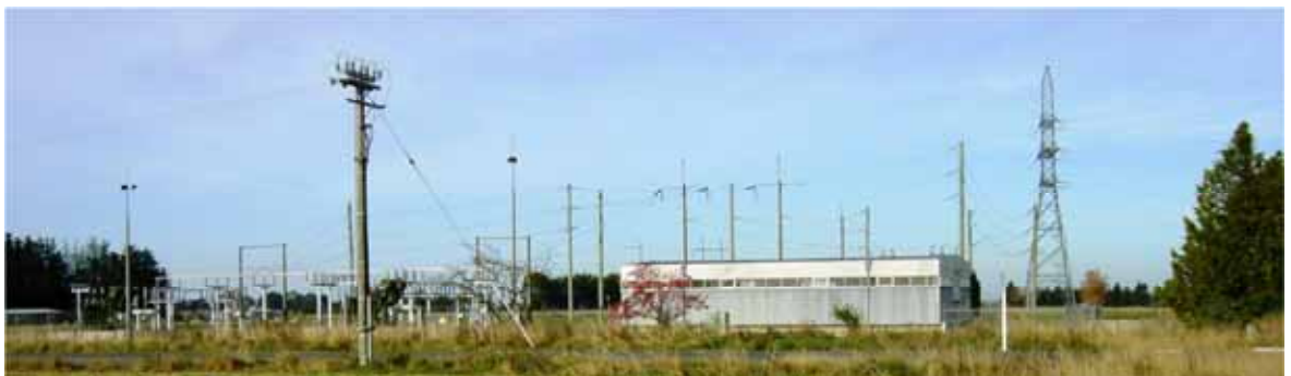
Figure 44 - Winton 66kV Substation
