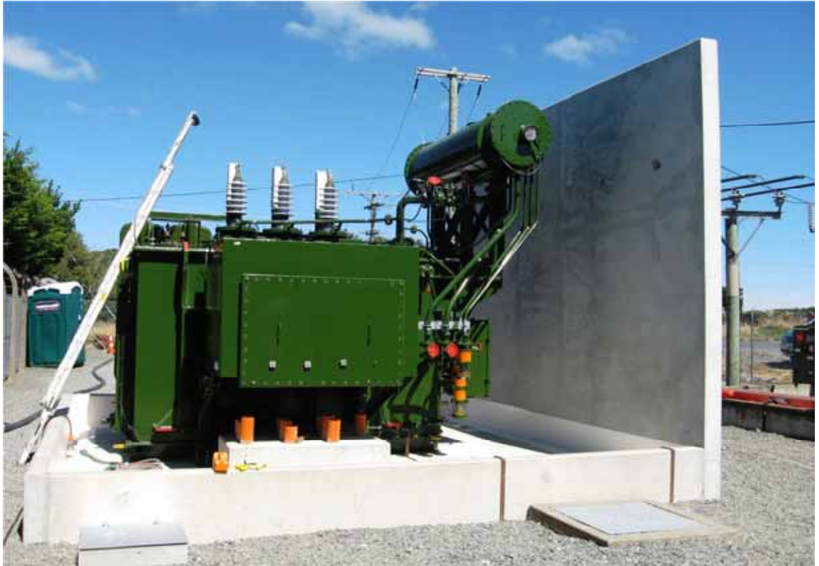
Figure 46 – New CGPT 33/11kV 6/12MVA Transformer
