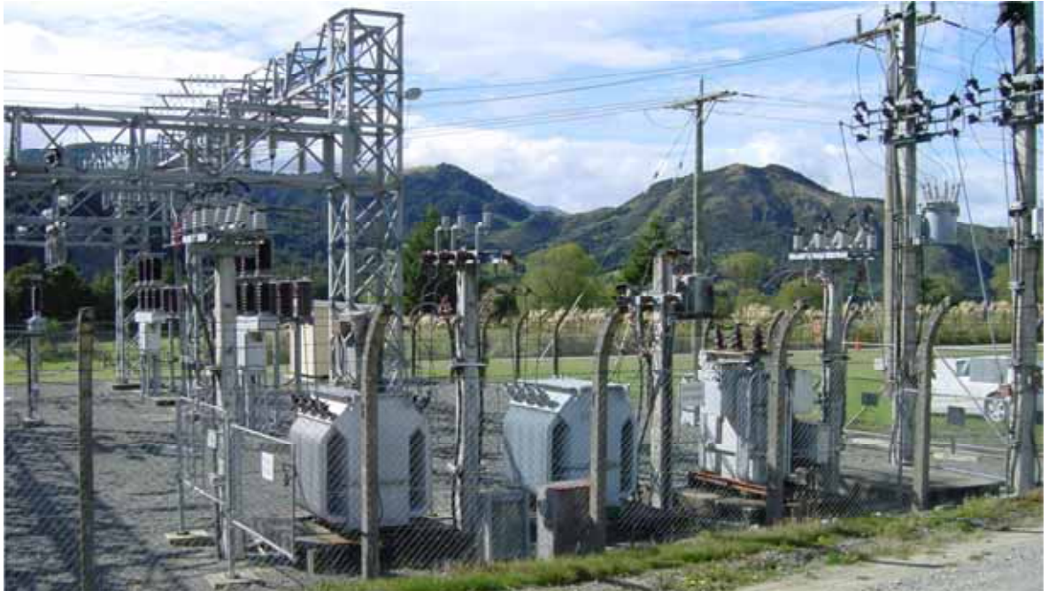
Figure 50 - Monowai Structure (6.6kV and 11kV equipment close to fence.)
