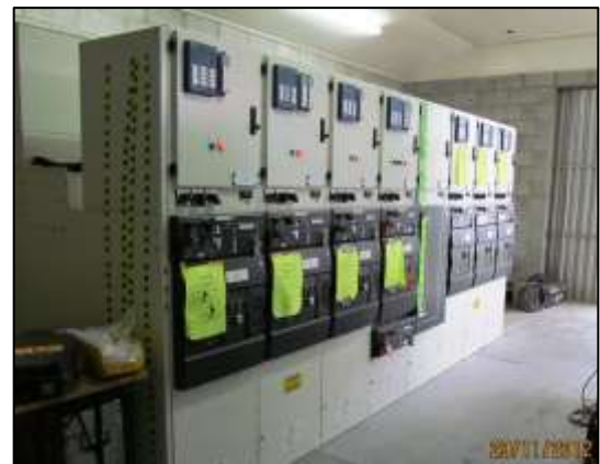
New switchboard at South Gore Sub
