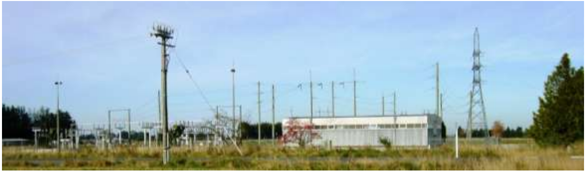
Figure 44 - Winton 66kV Substation
