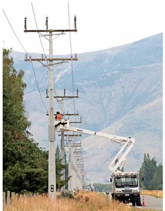
Delta Utility Services working on the Mossburn to Athol line upgrade
