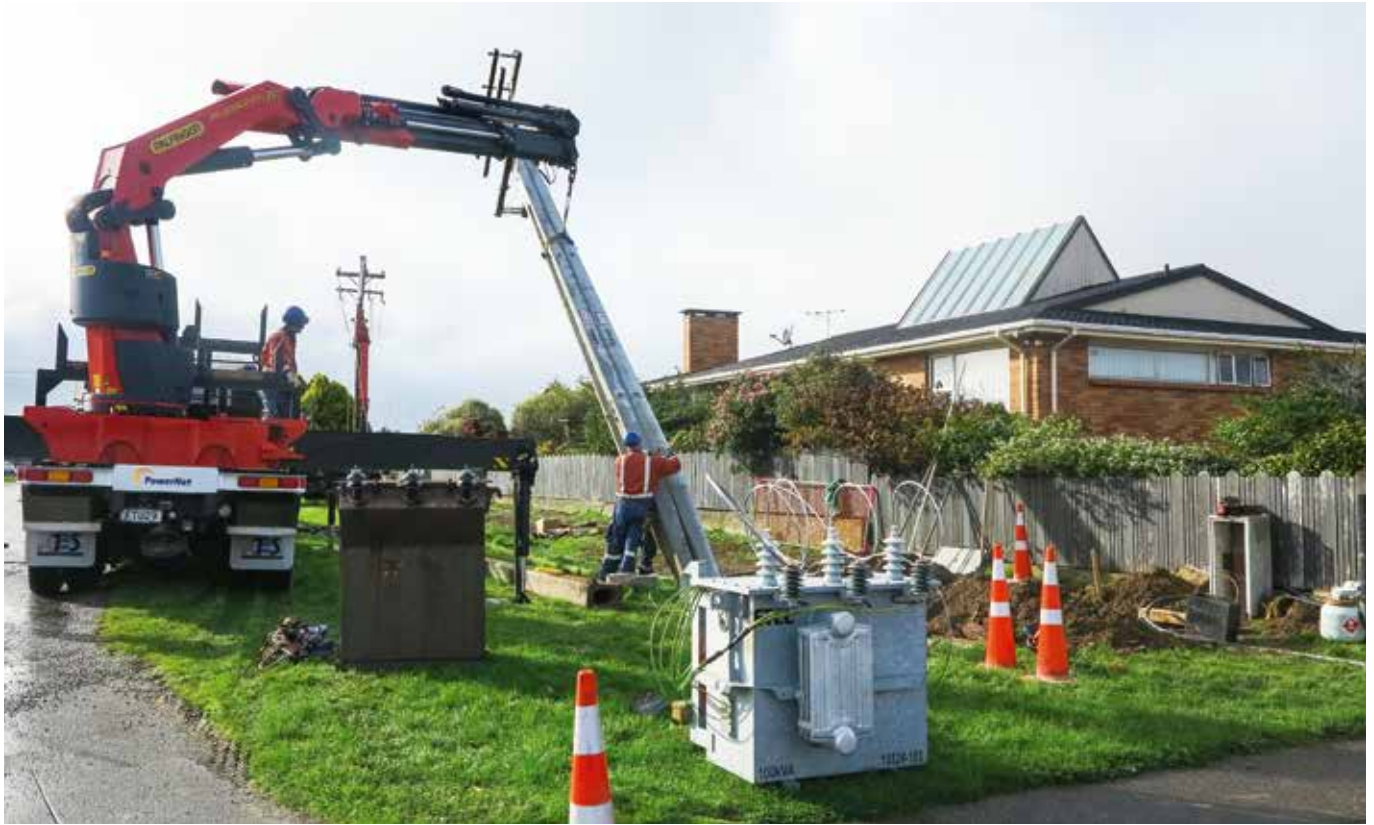
PowerNet Technical and Network Performance staff replacing a pole on the network
