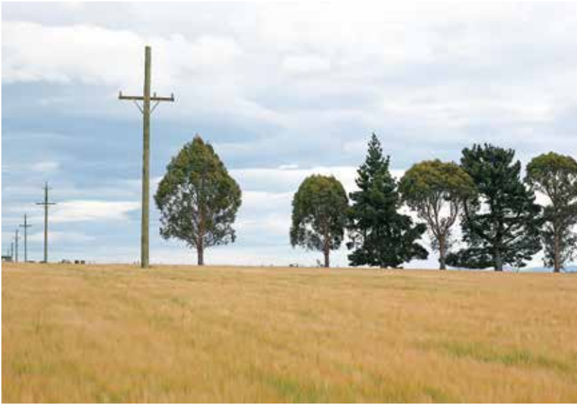
The new Mossburn to Athol 66/22kV line under construction
