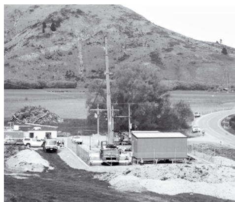
Athol Substation under construction
