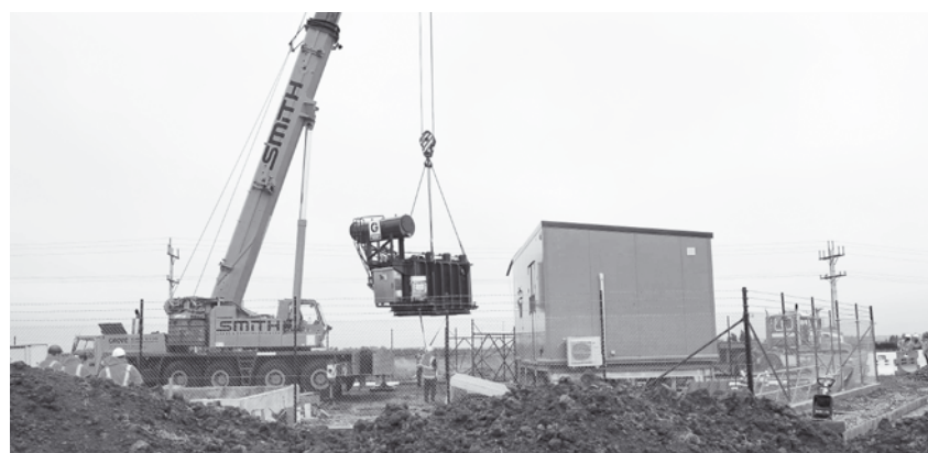
The 3/5MVA transformer being lifted on site at Hedgehope Substation
