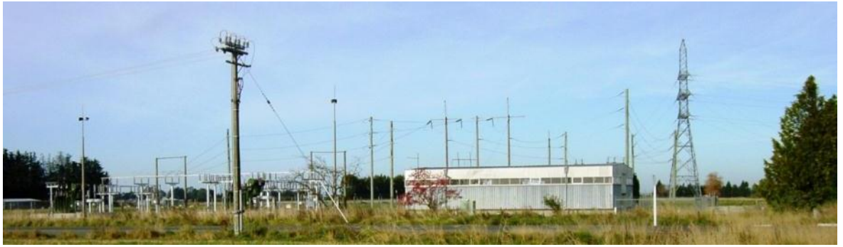
Figure 42 - Winton 66kV Substation
