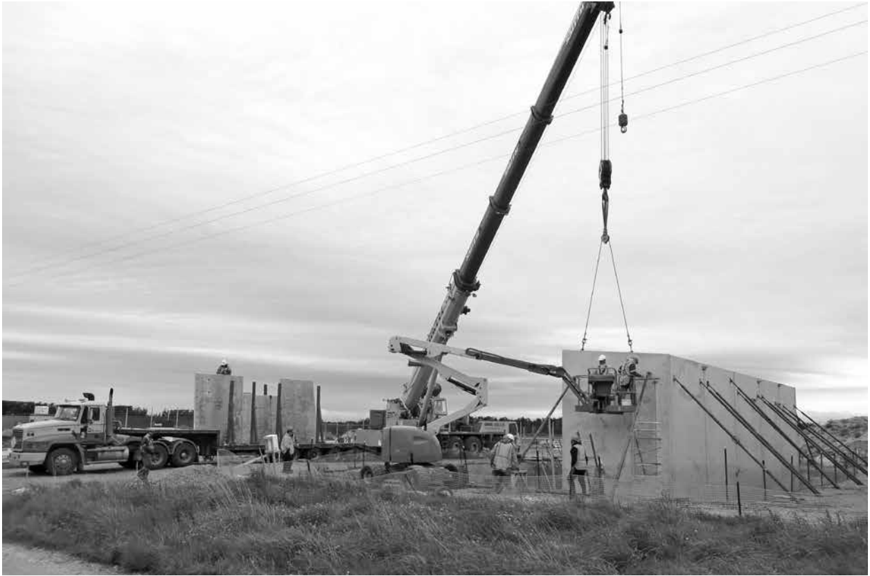
Colyer Road Substation under construction
