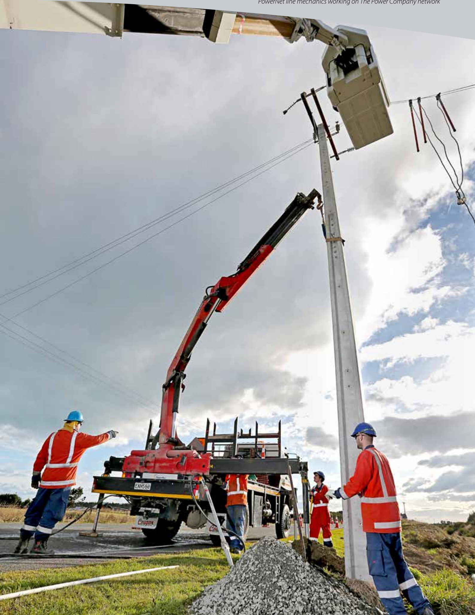
PowerNet line mechanics working on The Power Company network
