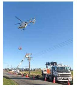
Staff from Otago Power Services installing the 66kV conductor on the new 66kV line
