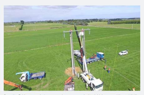
PowerNet Field teams replacing a two pole structure on the North Makarewa to Winton 66kV line
