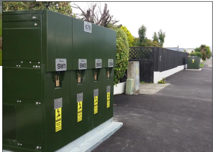
Underground Substation Replacement: 678 Herbert West of Carron
