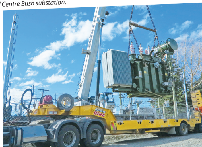
The 5MVA, 66/11kVA transformer being moved into position onto its concrete foundation inside the switchyard at Dipton substation.
