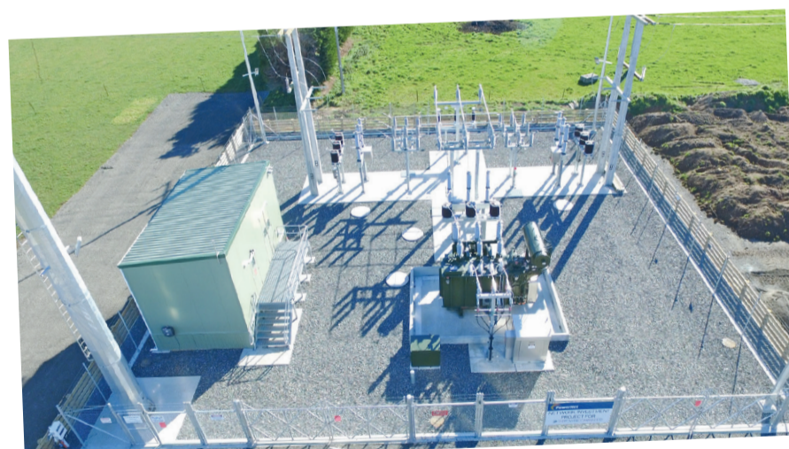
The completed Centre Bush substation.
