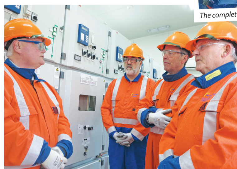
L-R: PowerNet project manager, Roger Scott and chief engineer, Roger Paterson with PowerNet directors Don Nicolson and Ross Smith inside the Centre Bush substation switch room.
