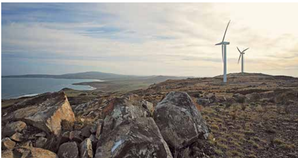
Flat Hill wind farm near Bluff.
