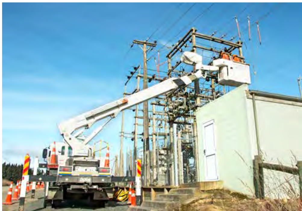
Port Molyneux substation, South Otago.
