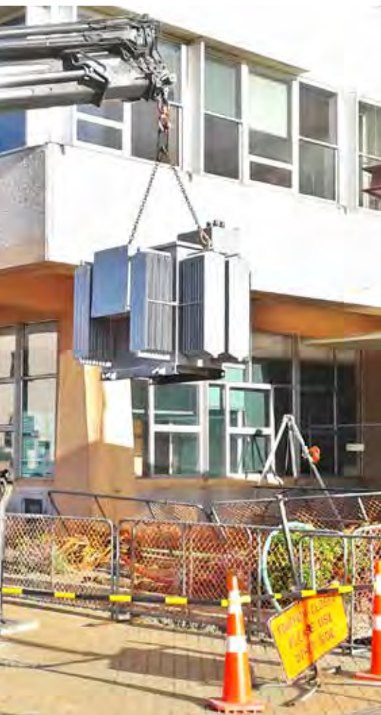
Evacuation work at the site of the civic administration substation, Invercargill.
