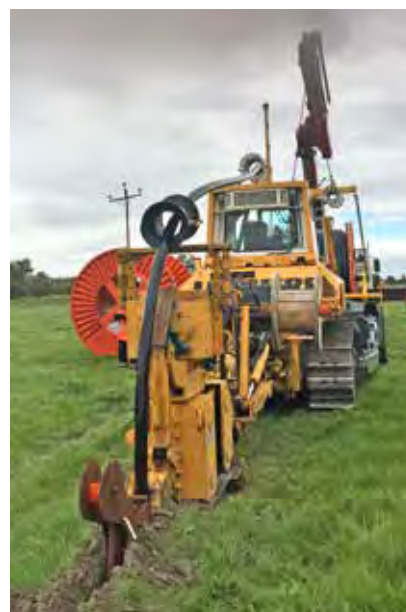
The mole plough used to install a cable at Clydevale.
