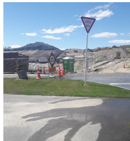
Installing the power supply to Clearview Subdivision.
