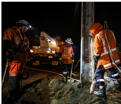
Pole replacement undertaken at night-time in Riverton.
