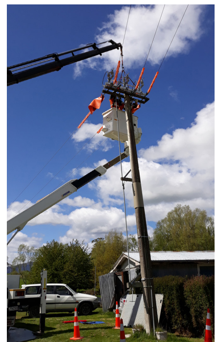
PowerNet teams working live-line, installing in-line isolators in the Balclutha township.
