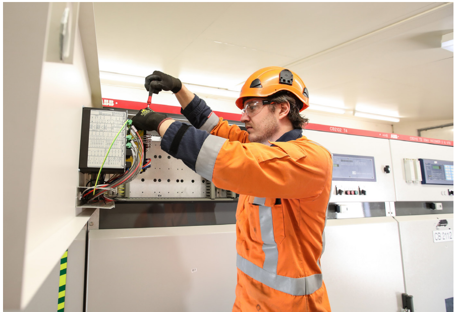
PowerNet apprentice substation maintainer Aaron McCallum working on replacing a protection relay at Edendale Zone substation.
