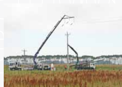
Live line work on the Catlins upgrade
