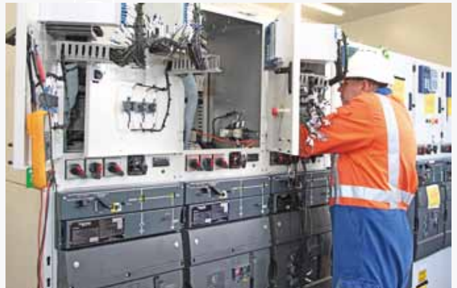
Arthur Everson from Transfield working on the Kennington Substation
