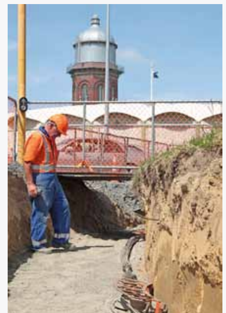
A contractor inspecting the new cable
