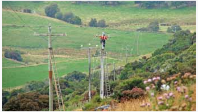
Otago Power Services line mechanic working on pole replacement on the Owaka to Tahakopa 11kV line
