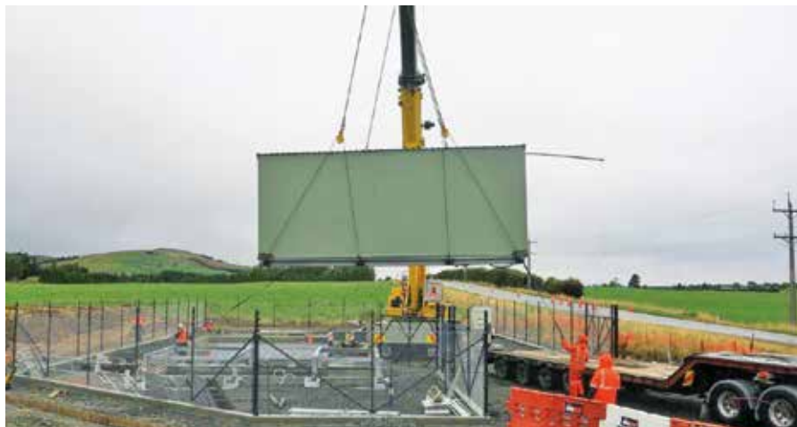
The new portacom being lifted on site at Hedgehope Substation
