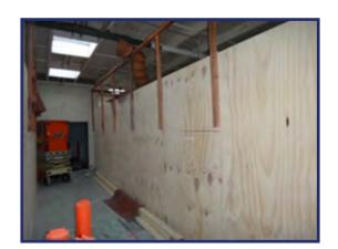
The physical barrier around the 11kV panels.
