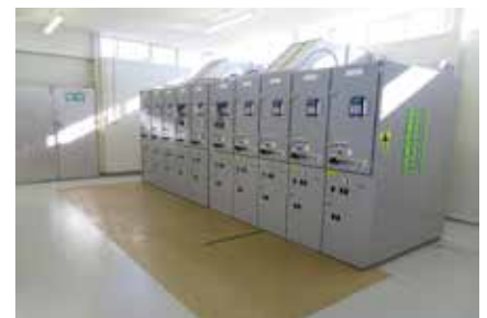
New Winton 11kV Switchboard
