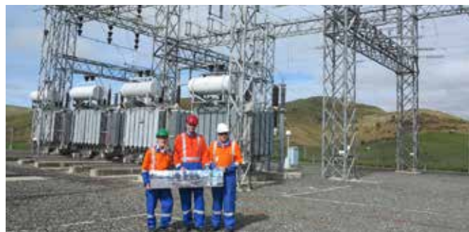
(L to R) Terry Jones (OtagoNet), Bevan Cooper (PowerNet) and Don Simms (Transpower) at the Palmerston Substation
