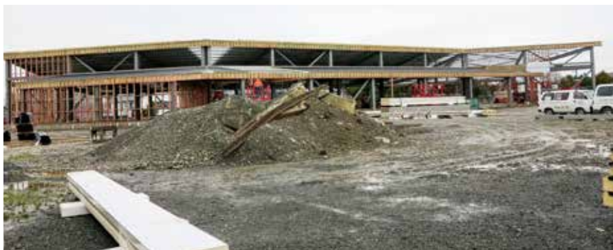
Contractors working on the PowerNet building on 11 August
