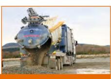
L-R: Skevington's vacuum truck extracts gravel from the holes before inserting the steel liner to prevent hole collapse.
