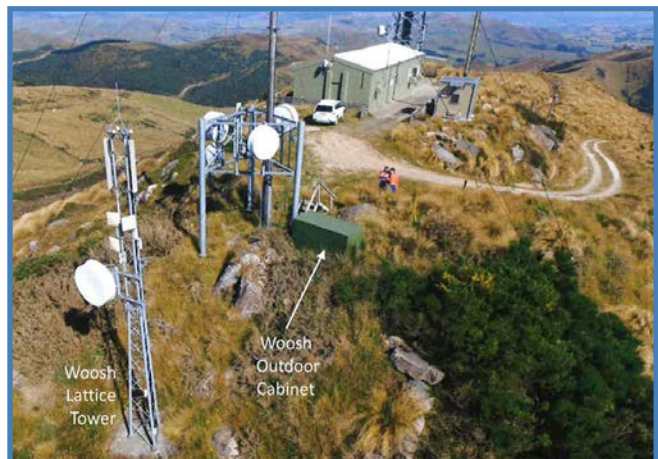
High Peak communications tower, West of Gore.
