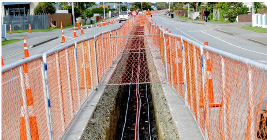
Stage two cable laying - Yarrow Street heading towards Racecourse Road
