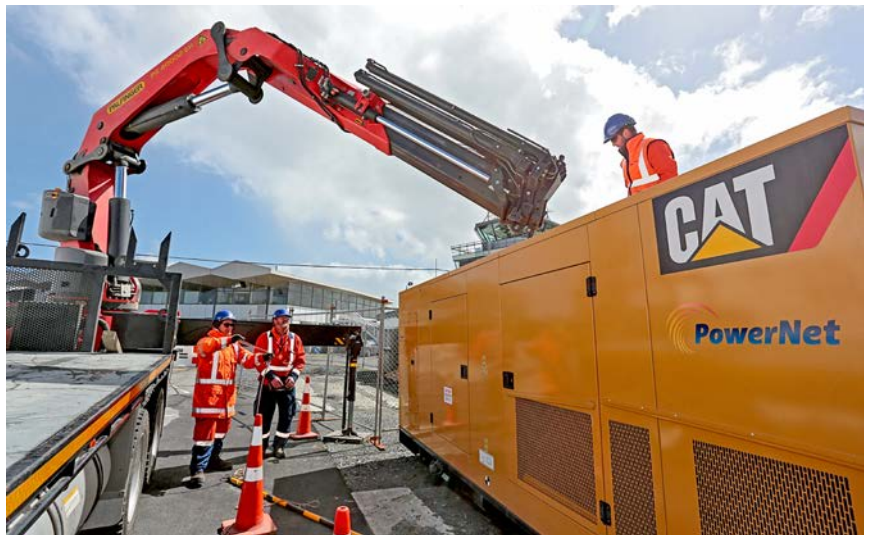
PowerNet staff Jordan Coutts, Allister Hitchcock and Jason Nicolson lifting the Caterpillar generator into place at the airport
