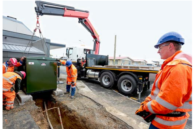
Phil Wilson and Ken McWilliam (Bond Contracts) with Peter Guise and Paul Barclay (PowerNet) placing the 750kVA transformer on site at Windsor New World
