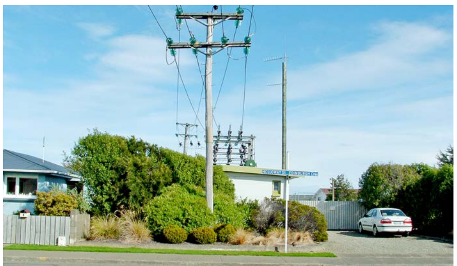
The existing Waikiwi Substation
