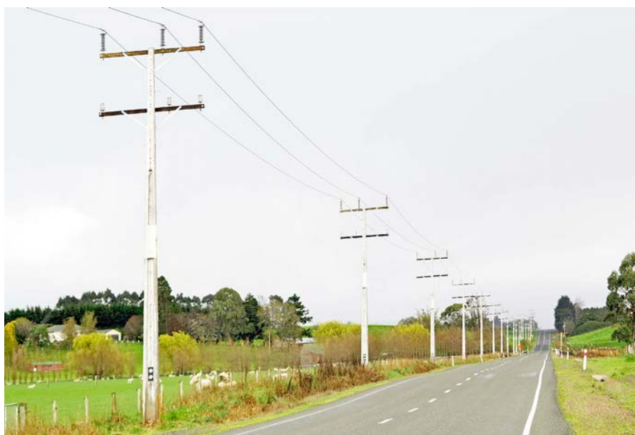
The Isla Bank to Fairfax 66/11kV Line
