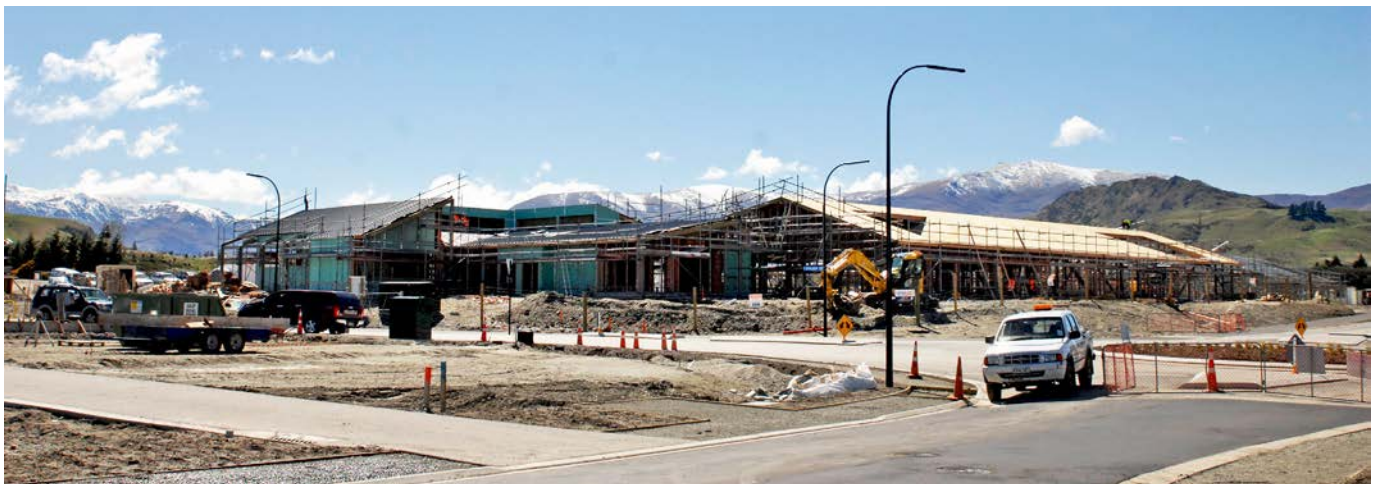
Shotover Primary School under construction
