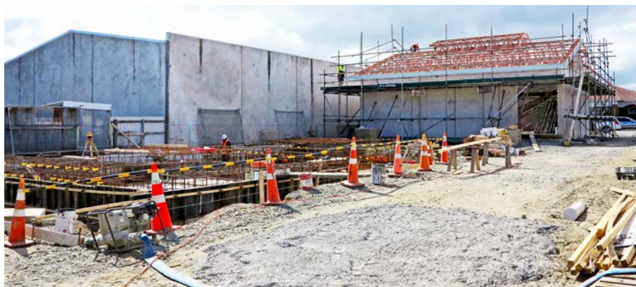
Foundations being boxed for the transformer
