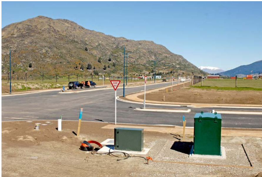
Eastern Access Road at Remarkables
