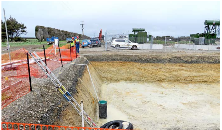
Groundwork on the Colyer Road Substation control room
