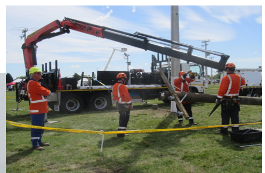
Above: The team working on the 'Hardware Build' category. This involved installing hardware and fittings on a softwood pole while being judged.
