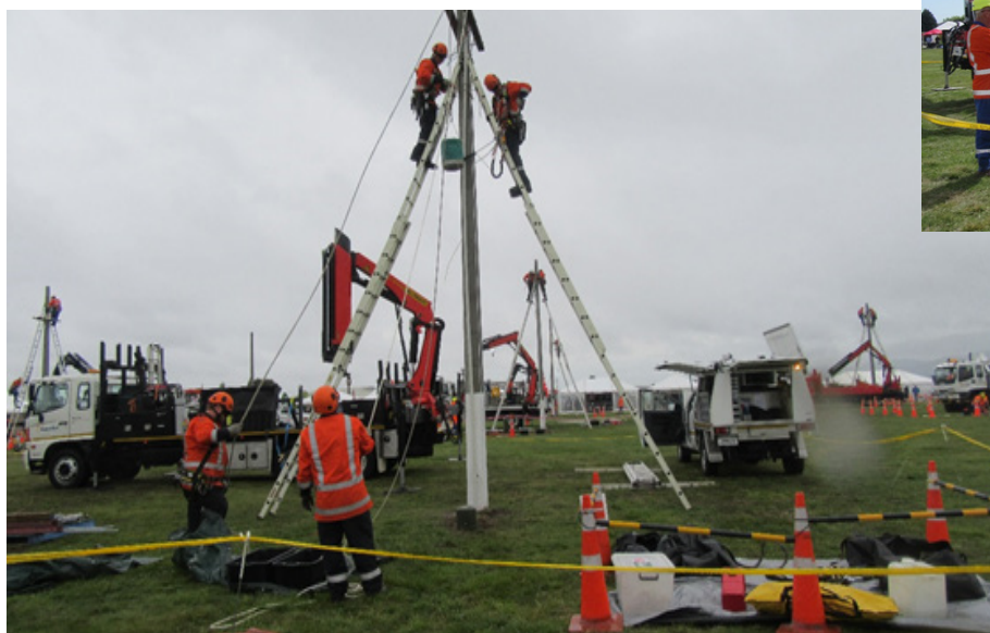
Above: The team working on the 'Hardware Build' category. This involved installing hardware and fittings on a softwood pole while being judged.
