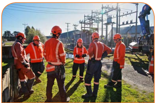
Chief operating officer, Michelle Henderson holding a team brief with the Balclutha team members at the Elderlee Street substation, Milton.
