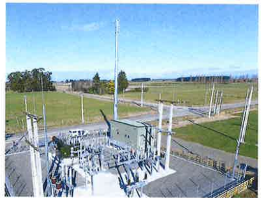
The upgraded Centre Bush substation.
