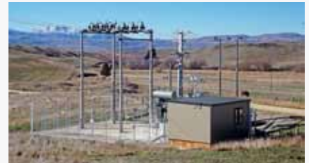
Before and after photos of Waipiata Substation
