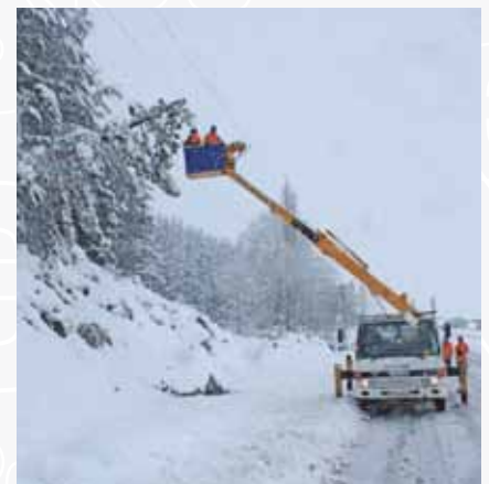
Power Services fixing lines on the network
