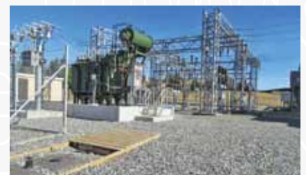
Contractors lifting the new 66/11kV transformer on-site
