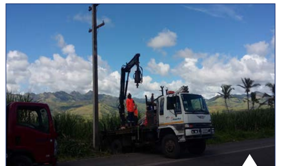
The PowerNet crane truck working on the Fijian network
