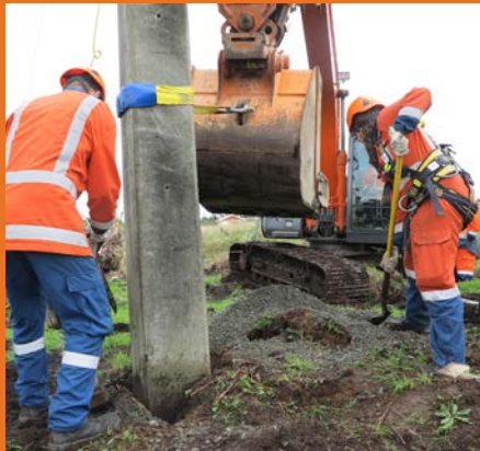
Left: Gene Brookland and Ione Pau compacting the ground around a pole Right: Line restringing preparation across State Highway 1
