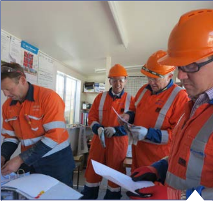
Left to right: Phil Johnson (Decom), Don Nicolson, Doug Fraser (PowerNet Directors) and Jason Franklin (PowerNet Chief Executive) being inducted onto the Waikiwi Substation construction site.
