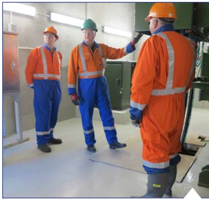
Left to right: Tim Brown, (PowerNet) Peter Leith (Decom) and Alan Harper (PowerNet Director) in the enclosed T1 transformer room
