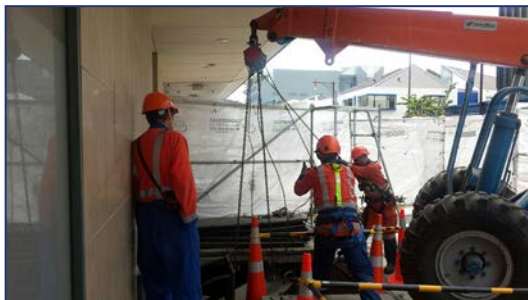
The old 1962 750kVA transformer being lifted above ground and the new 1,000kVA transformer behind The Southland Times
