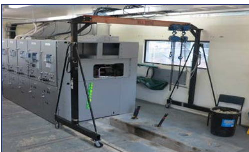
Left: The old switchgear is removed, a concrete pad laid and the new switchgear (right) placed into position
