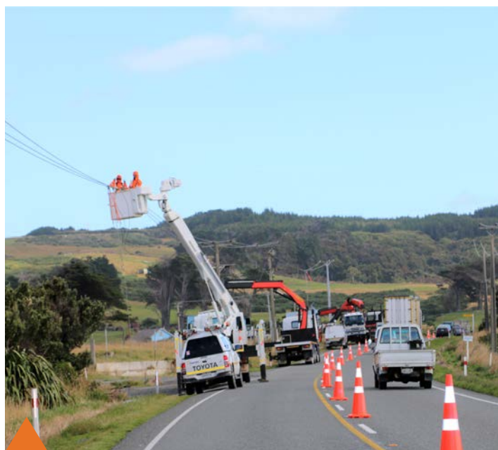
PowerNet distribution line mechanic teams working on the pole upgrade near Bluff.
