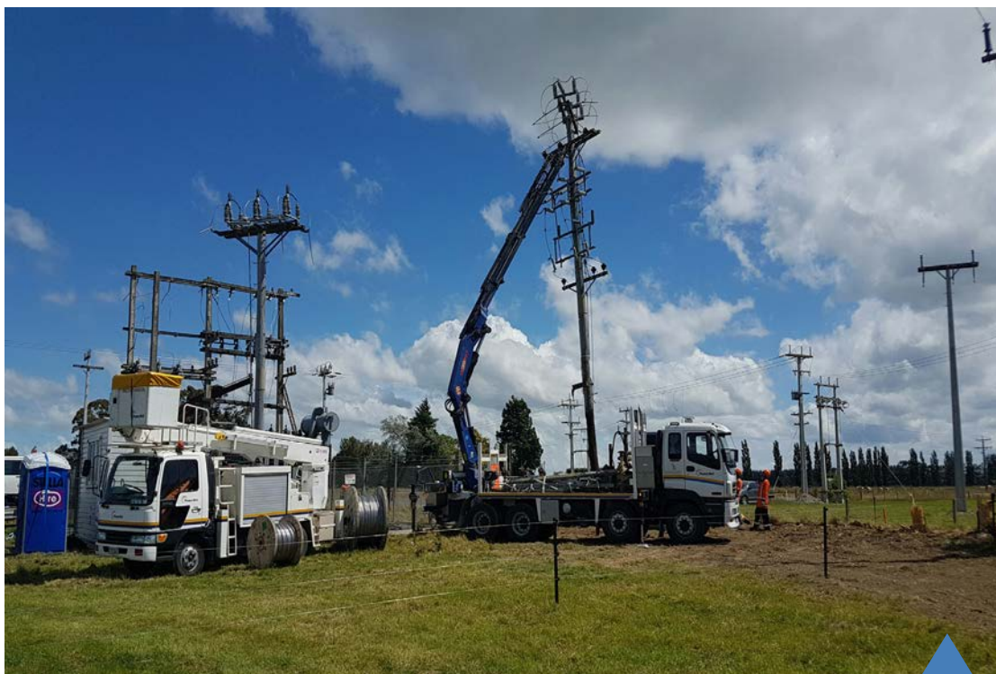
PowerNet's distribution line mechanic team working on the Centre Bush Substation upgrade.
