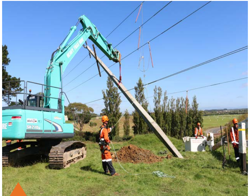
Above and below photos show pole replacements in Makarewa.
