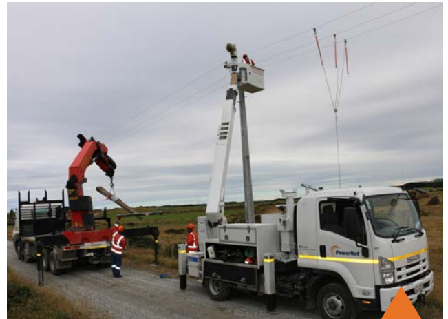
PowerNet's Onslow distribution line mechanic team working on replacement poles on Casey Road in Otaru.
