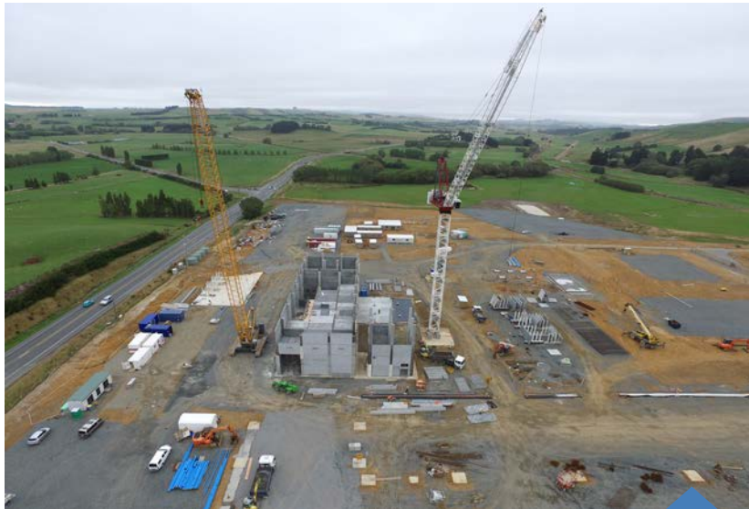
A drone photo of the construction site at Matura Valley Milk. (Photo supplied by Southroads).
