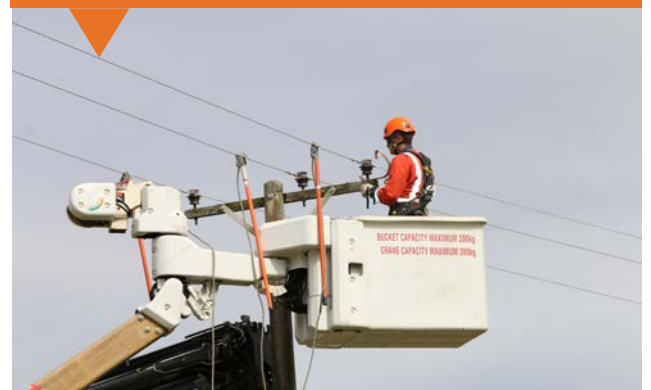
PowerNet's Onslow distribution line mechanic team working on replacement poles on Casey Road in Otaru.
