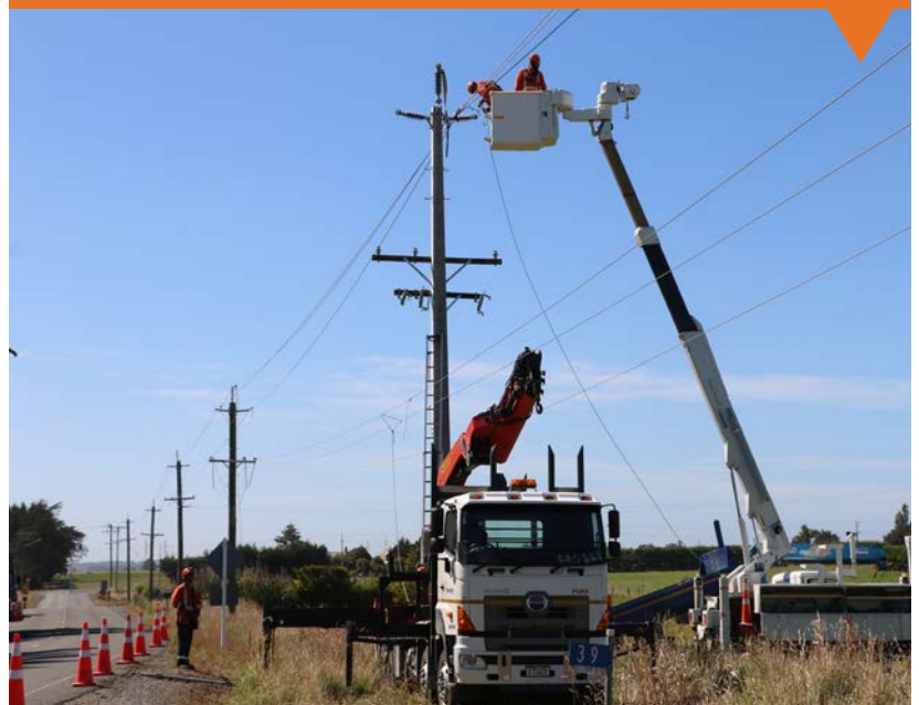
Above and below photos show pole replacements in Makarewa.
