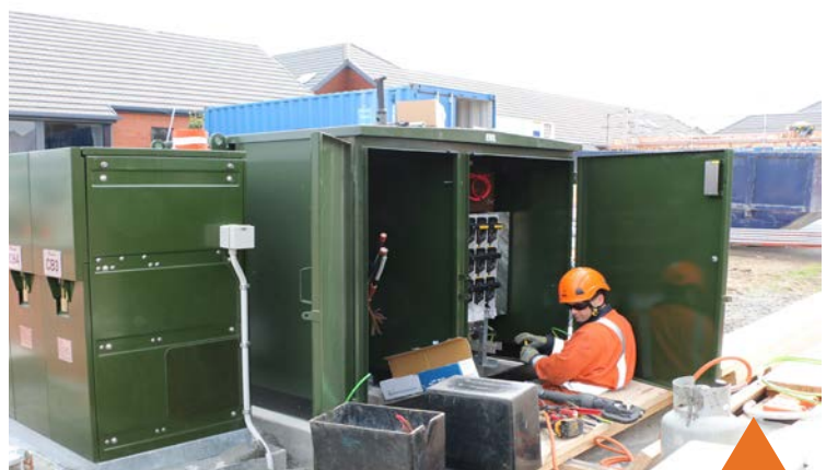
PowerNet's substation maintainer, Brad Templeton working on the 750kVA transformer
