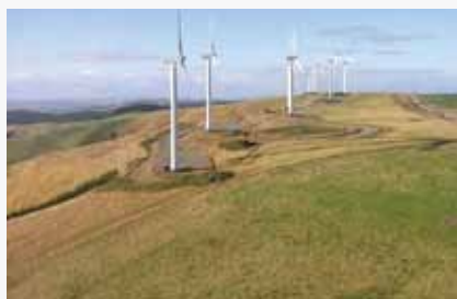
Mt Stuart Wind Farm
