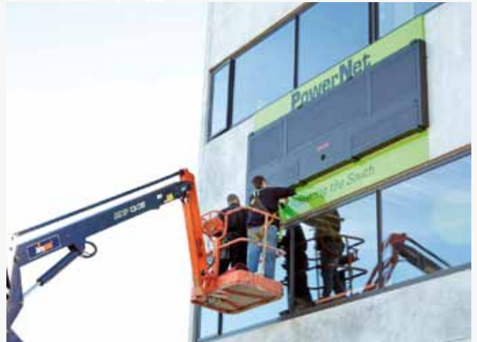
Vital Signs Team erecting the PowerNet signage at Southland's Rugby Park
