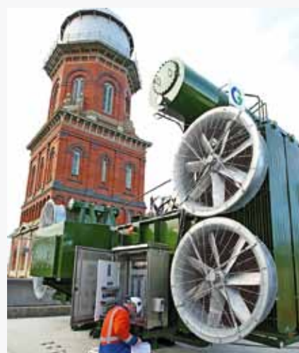
Jeff Carmody working on the 33/11kV transformer at Doon Street substation
