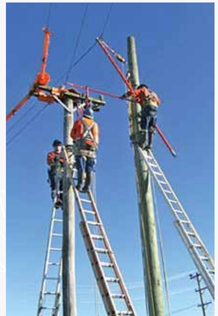
Left to right; Shane Lawson, Joseph Reti and Lance Harris replacing an 11kV pole on the training line
