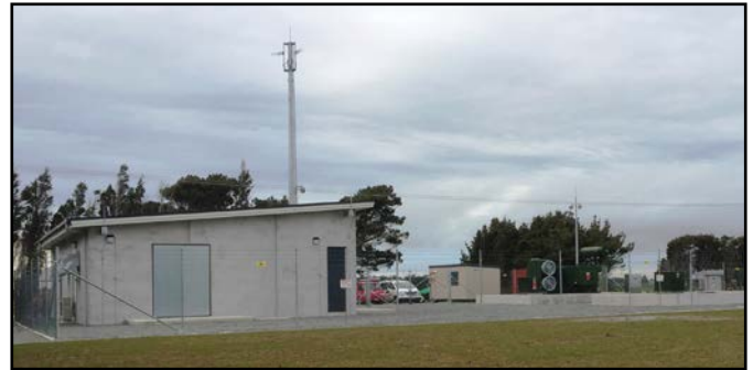
Colyer Road Substation
