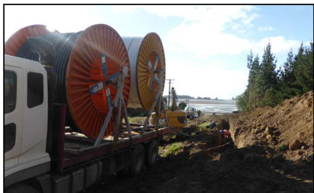
Staff from Otago Power Services laying cable
