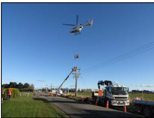
Staff from Otago Power Services installing the 66kV conductor on the new 66kV line
