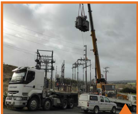
The PowerNet team working on the Clydevale Substation
