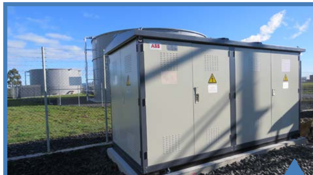
The weather proof housing for the indoor 33kV Ring Main Unit
