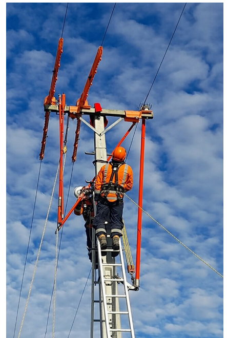
In-house live-line training.
