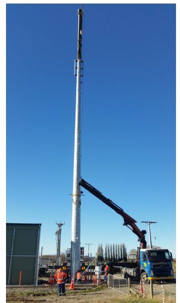
The Communications tower being installed at the Centre Bush Zone substation.
