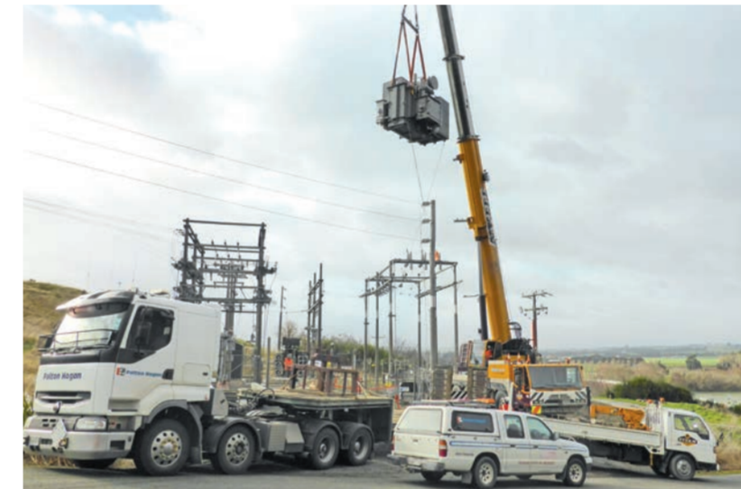
The 5MVA transformer being lifted on-site
