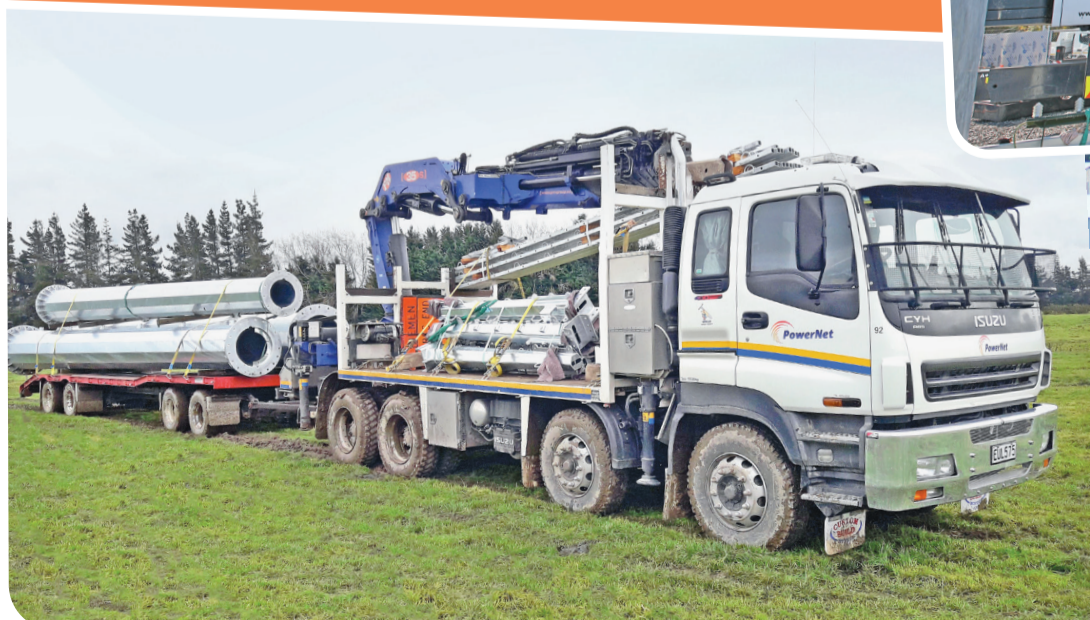
One of the four 38m steel towers being delivered to the Oreti River site to be installed.
