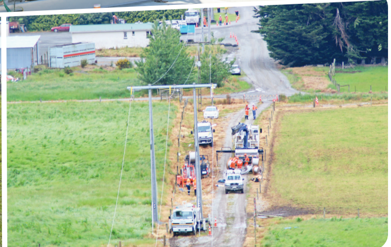
PowerNet staff and contractors installing the 66kV conductors across the Oreti River.
