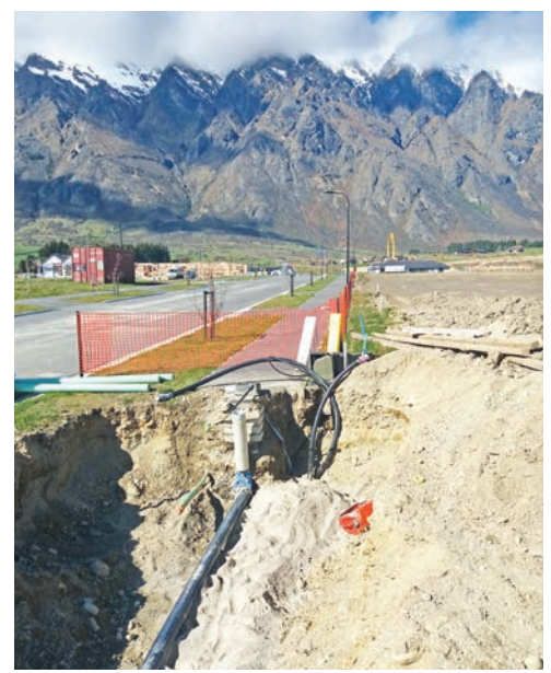
Cable trenching at Hanley's Farm.
