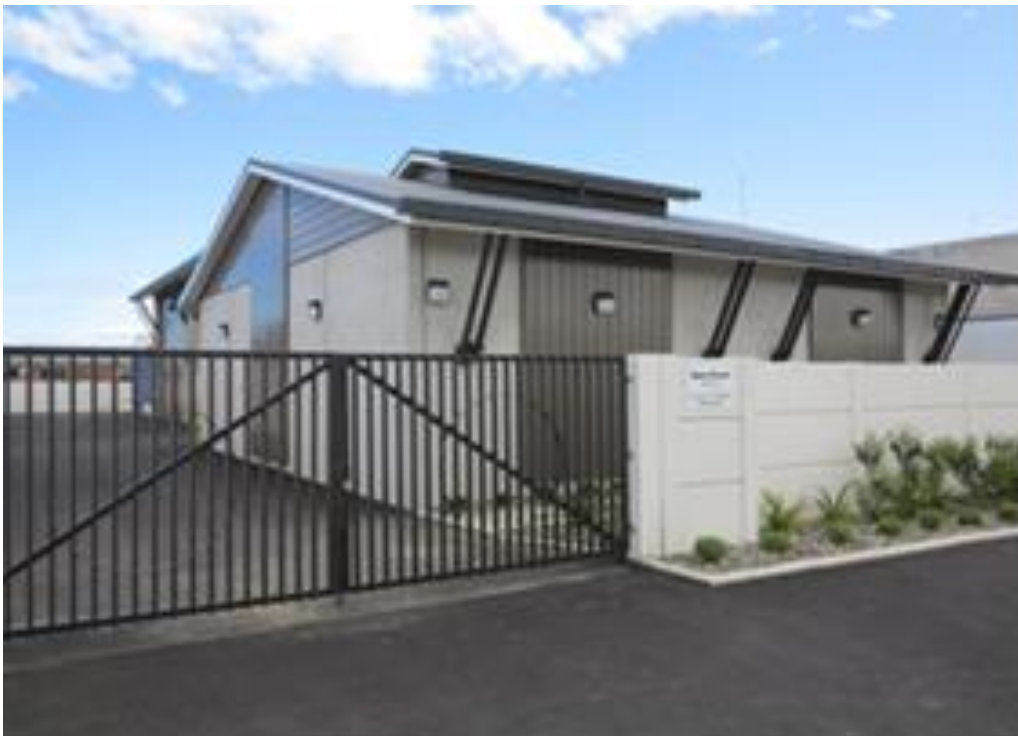
Spey Street Substation
