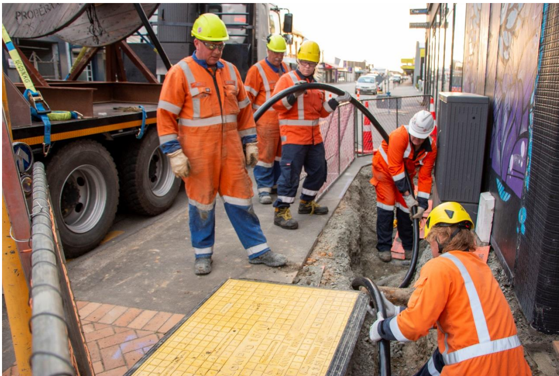
PowerNet and BCL pulling new cables to upgrade the network for the Langlands Hotel complex
