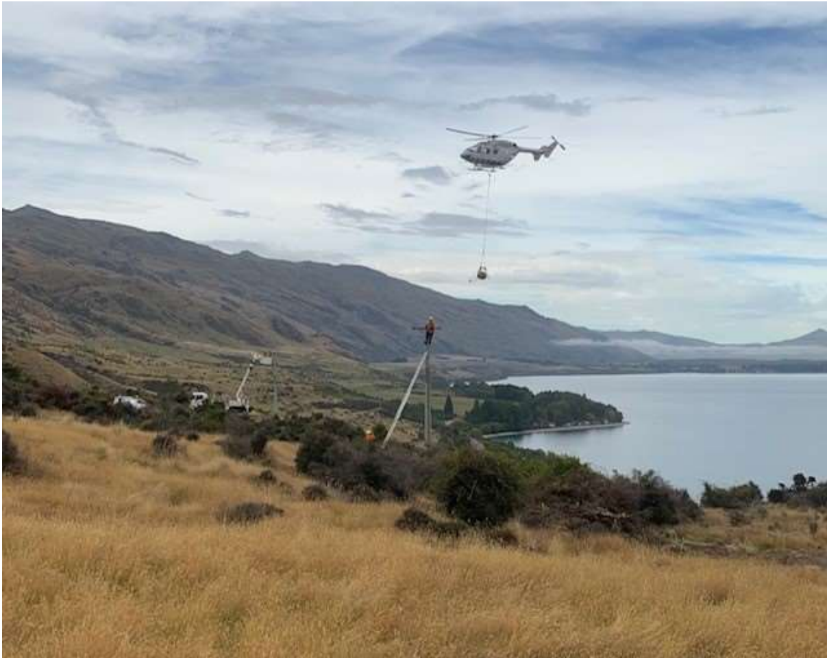
Helicopter Conductor Stringing - Kingston
